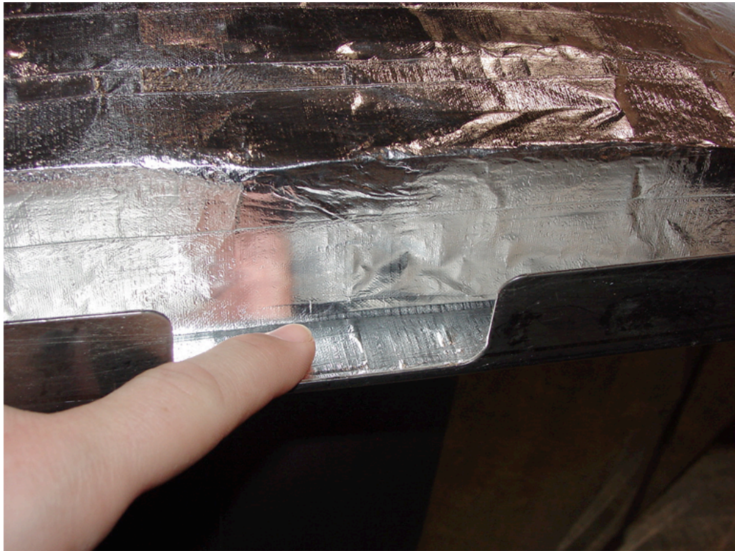
Figure 14. Taping of the Plenum (Bottom).
