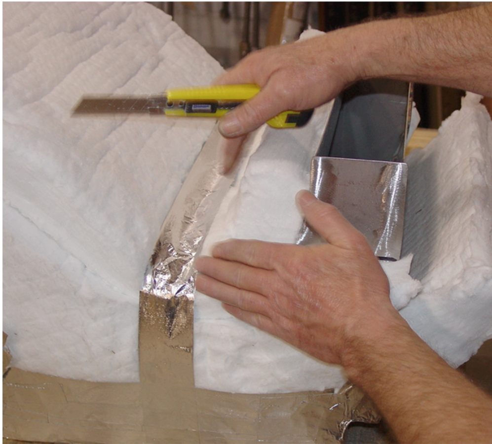
Figure 26. Taping Bend to Keep it in Place (Sheet 1 of 2).
