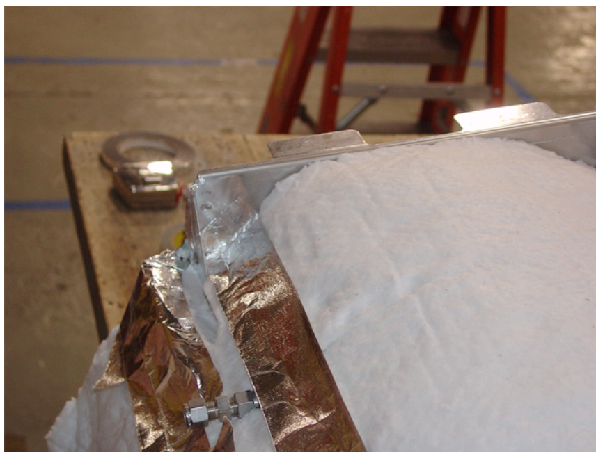
Figure 19. Taping Down the Insulation (Sheet 2 of 2).
