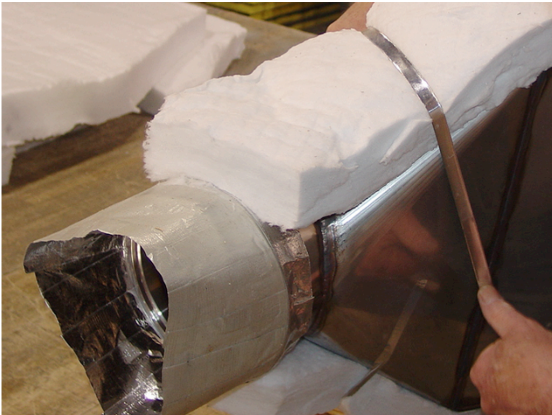
Figure 15. Preparing Insulation for Taping (Sheet 2 of 2).
